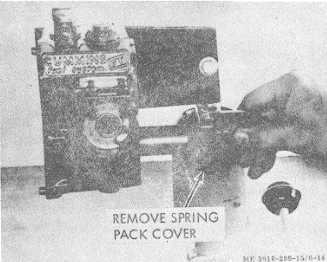
Figure 3-15. Spring pack cover removal.
